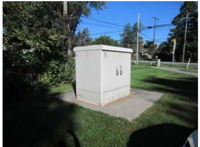
Pad Mounted Transformer
