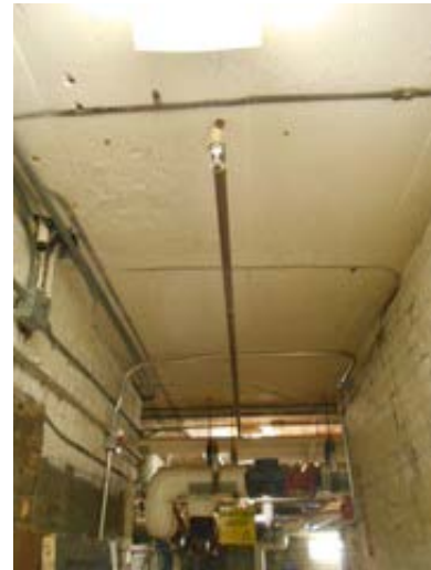
Compliant Suppression System-Boiler Room
