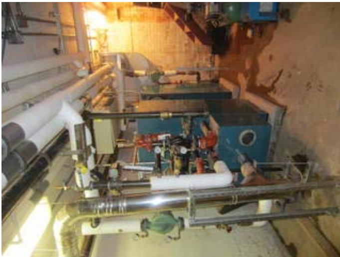
Natural Gas Fired Heated Water Boiler
