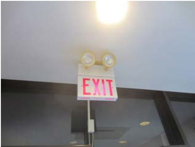
Exit Sign with Emergency Egress Lighting
