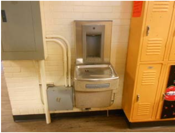
Electric Water Cooler
