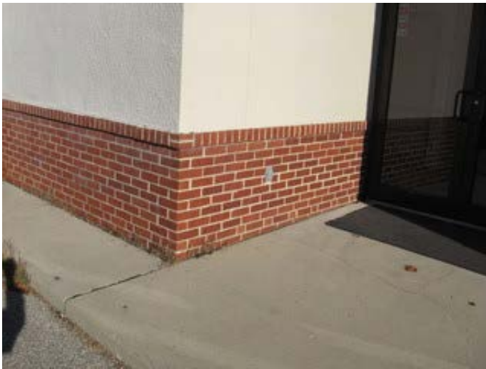
Brick Wainscot and Stucco Wall
