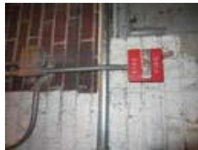
Fire Alarm Audible Horn and Strobe Indicating Device
