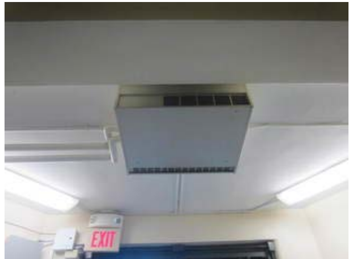
Heating Water Cabinet Heater
