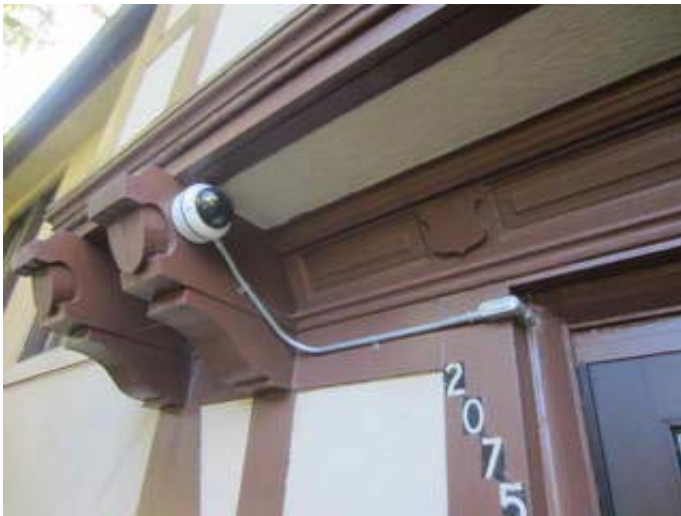
Security System CCTV Camera
