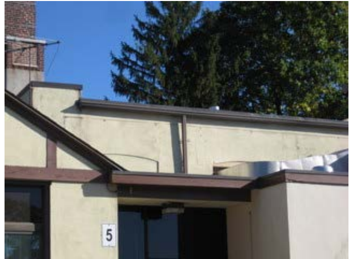
Flashing at Low Slope Membrane Roof
